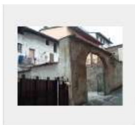
Casa Via Monte Grappa 4 Lumezzane (BS)
