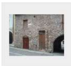
Casa Via Home 58 Lumezzane (BS)
